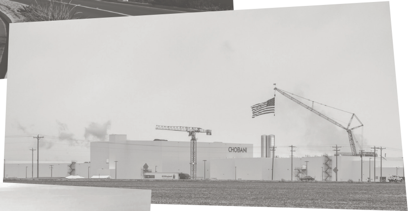
Chobani Production Facility, Twin Falls, ID
