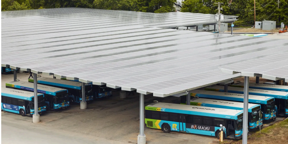
Figure 2. The Brookville Smart Energy Bus Depot combines solar and battery storage to power electric buses in Maryland
