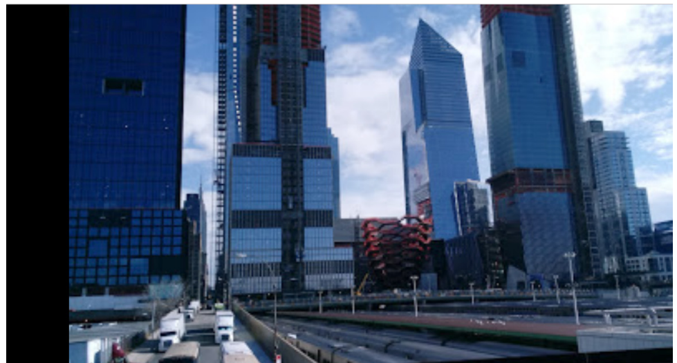
Figure 3: Hudson Yards under Construction above MTA Storage Yard, February 2018
