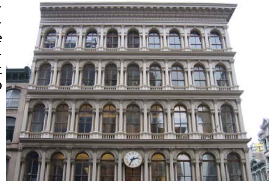
The E.V. Haughwout Building is one of many cast-iron buildings in SoHo that would have been lost to the LOMEX.
